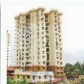
ORIENTAL GARDENS - SOUTH Kaloor
