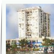
BAYPRIDE TOWER Marine Drive
