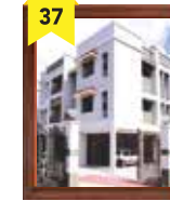
BLOSSOM APARTMENTS Sakthan Thampuran Nagar, Trichur
