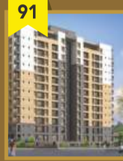
91 GARNET Off Mavoor Road, Calicut
