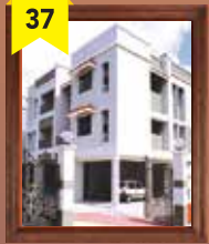
37 BLOSSOM APARTMENTS Sakthan Thampuran Nagar, Trichur
