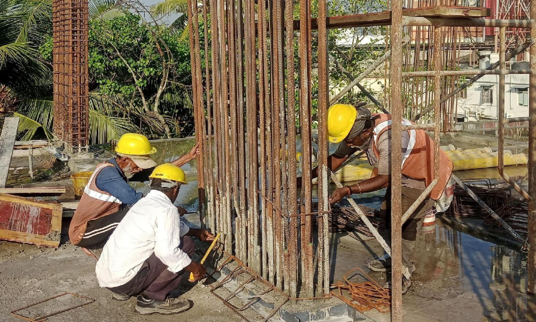
3rd floor column reinforcement
