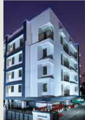
VARMA MAALIKA II LUXURY APARTMENTS 38 JUNCTION, TRIPUNITHURA
